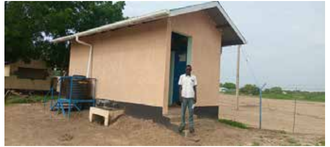
Constructed latrine @ Save The Children in Abyei Administrative Area.
